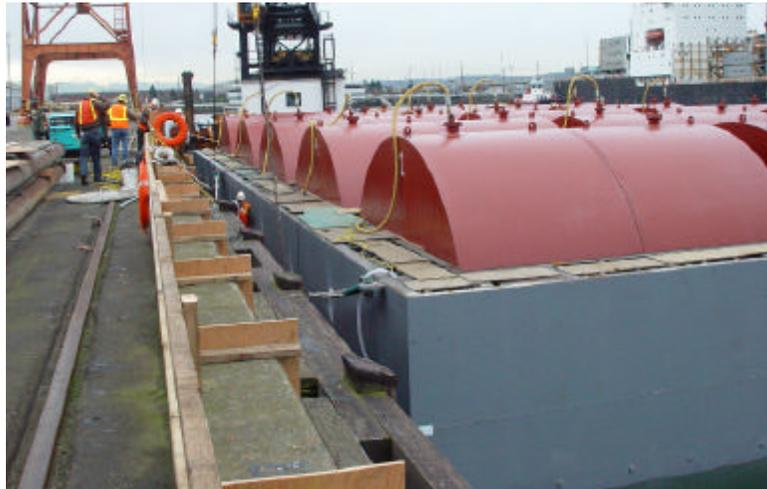
**Figure 7 Cutting Edge and Domes at the Yard, Under Construction**
