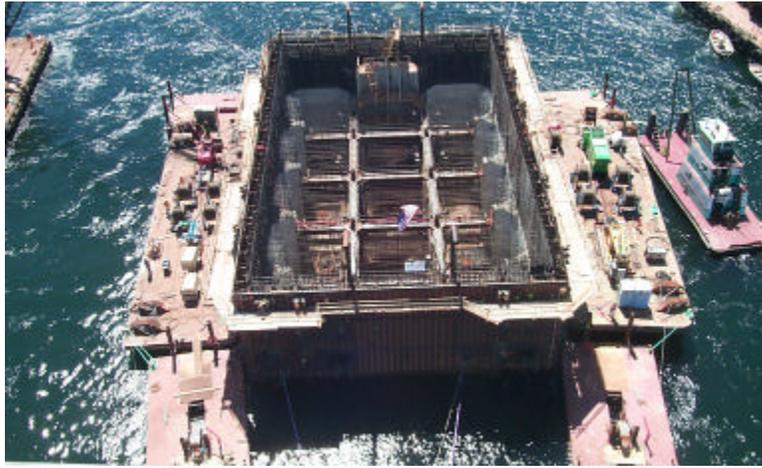
**Figure 10 Caisson Assembly during Floatout**
