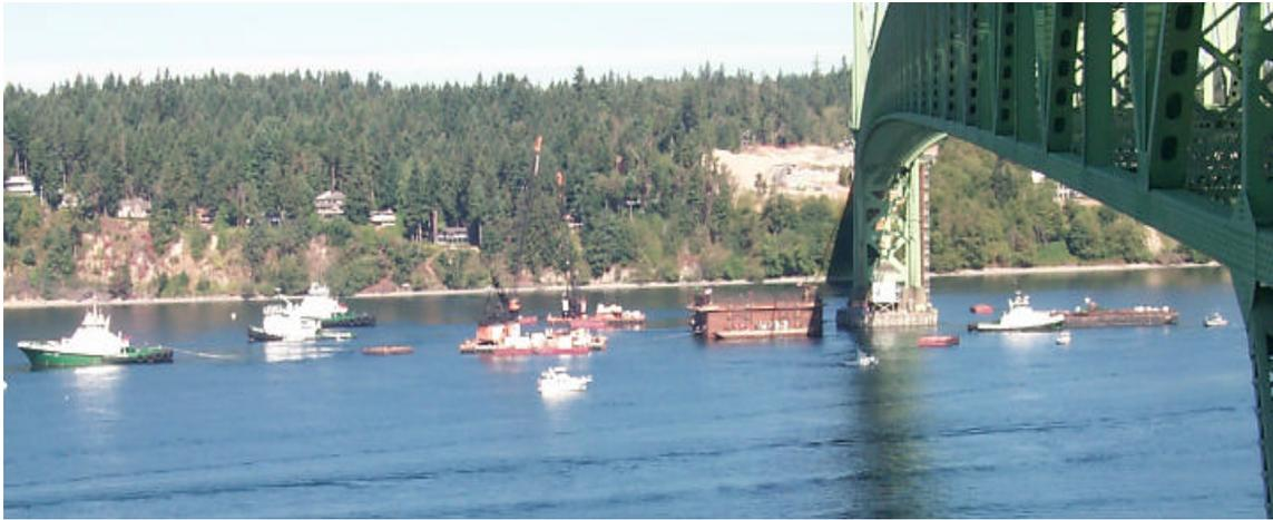
**Figure 8 Towing of Caisson to Site**
