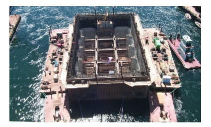
Figure 10 Caisson Assembly during Floatout
