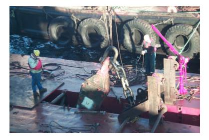
Figure 12 Making up Chain to Block
